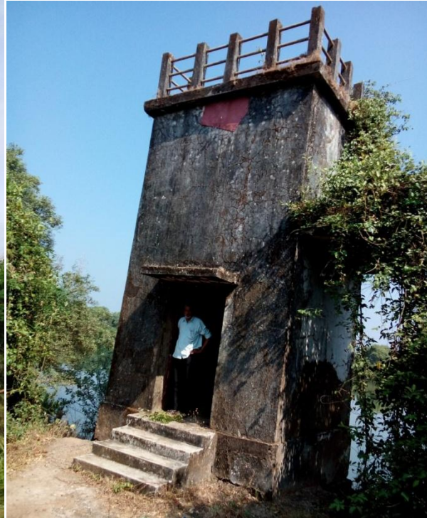
Light House at Maina
